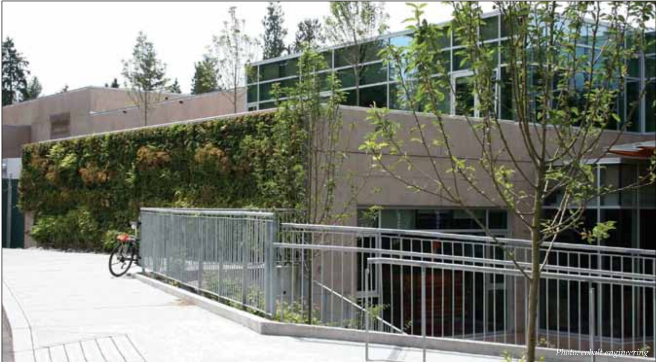
Figure 14: Reducing solar intensity with a green wall (Aquaquest at Vancouver Aquarium)
