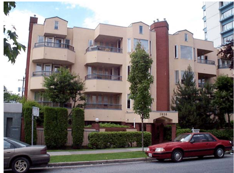
Apartment Building to the south of 911 Denman
