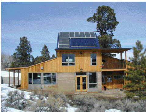
Examples of evacuated tube panels
