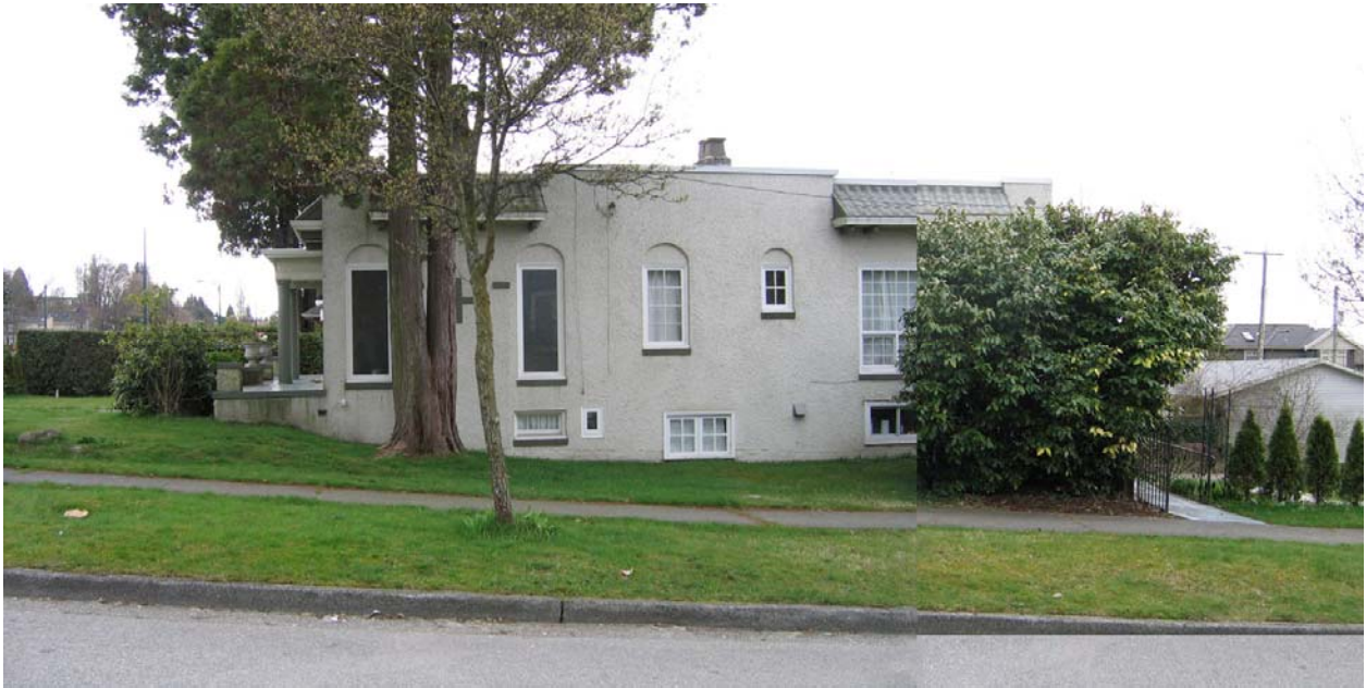
3409 Arbutus Street - North Side of the Heritage Building (current condition)
