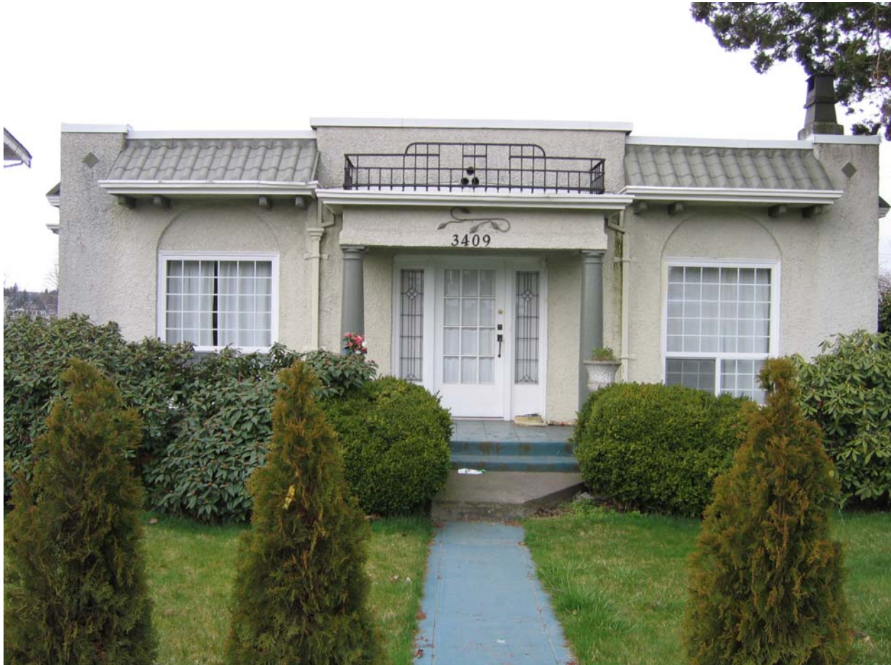
3409 Arbutus Street - Front of the Heritage Building Facing Arbutus Street (current condition)
