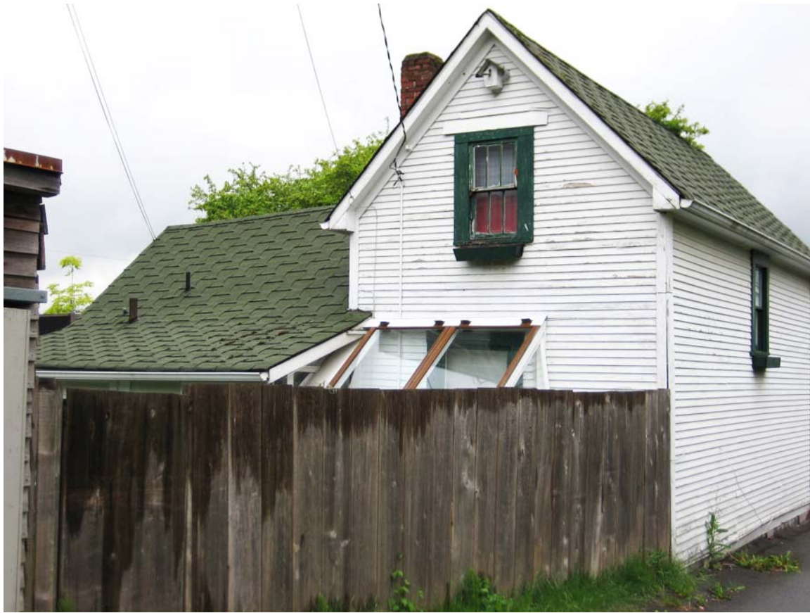
212 East 38 th Avenue- Rear of the Heritage Building along the Lane
