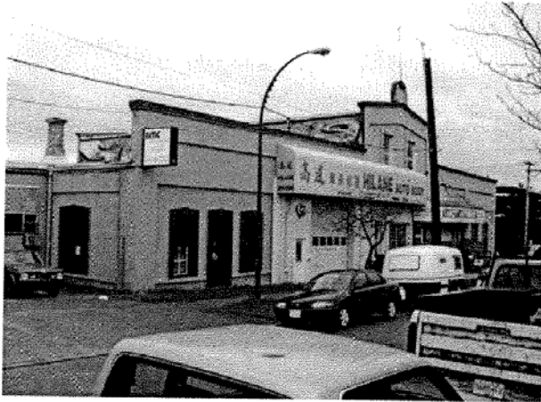
Front of the Heritage Building from 7 th Avenue
