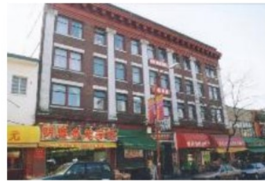
3 254-262 E Pender Shon Yee Benevolent Association (May Wah Hotel) Year Built: 1914 Heritage Category: B
