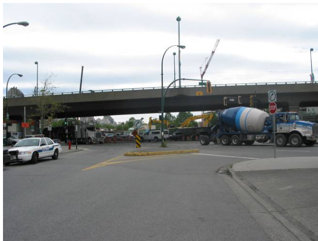
Figure 3: Westbound 5 th Avenue approaching Cambie Street and 2 nd Avenue
