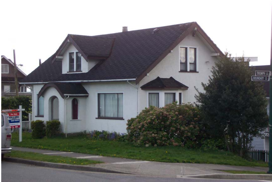
125 Boundary Road - North-east corner
