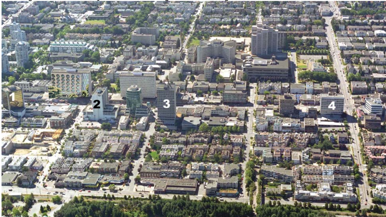
Figure 3 - Broadway Corridor looking south showing the four towers built in the 1970s
