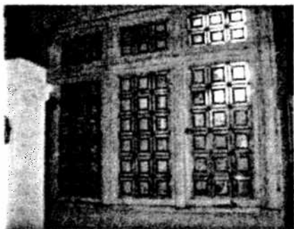
Photo 31: Staircase stained glass casement window, north elevation
