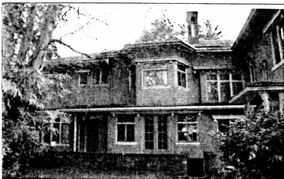
Photo 2: North elevation with northern annex on right
