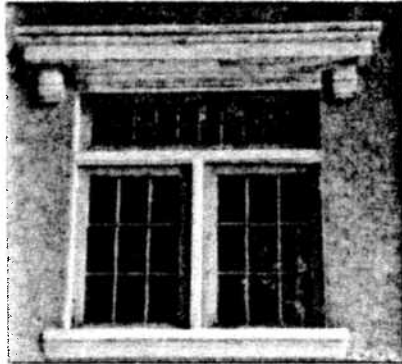
Photo 18: Original casement window with flat lintels over
