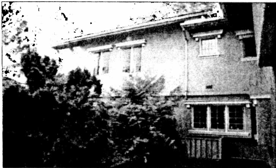
Photo 10: Northern annex, west façade
