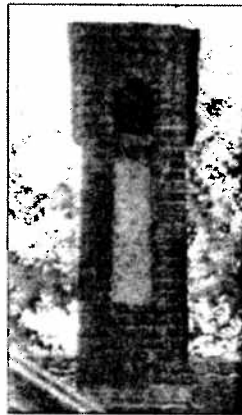
Photo 16: Original chimney with corbelled brick
