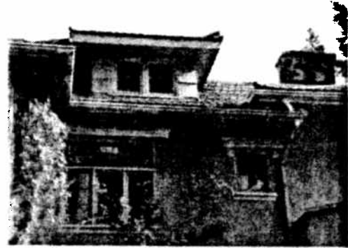
Photo 13: Differing eave heights with shed dormer above
