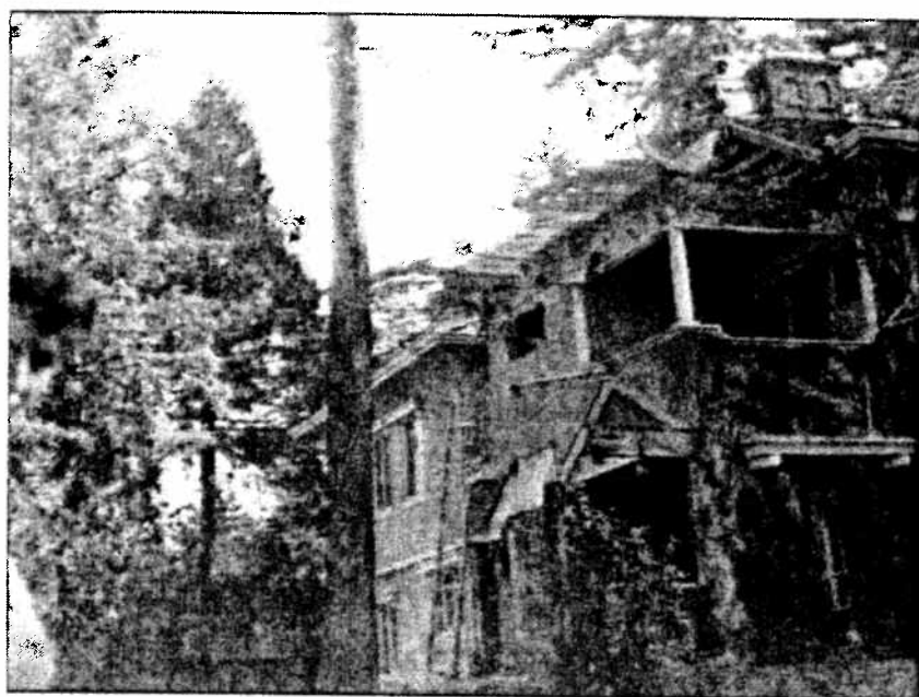
Photo 9: Demolition of conservatory buildings [Killam Family photograph]
