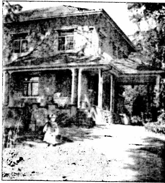
Photo 6: View of original east elevation and porte-cochère [Killam Family photograph]
