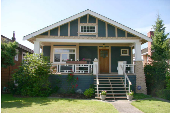
Front/north elevation which will include the addition of an entrance for the garden suite.
