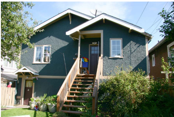
Rear/south elevation which will be added on to.
