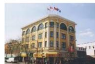
11 525 Gore Chinese Nationalist League of Canada (Kuomingtang Building) Year Built: 1920 Heritage Category: A
