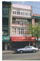
2 27 E Pender Wong's Benevolent Association (Han Shen Building) Year Built: 1910 Heritage Category: B
