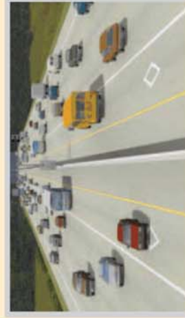
Pre-design concept proposes 3 lanes in each direction for general commuters and goods movers and one lane for HOV between Vancouver and Surrey
