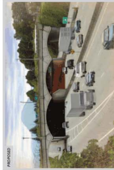
PROPOSED Cassiar Connector looking west, after improvements, with three lanes in each direction
