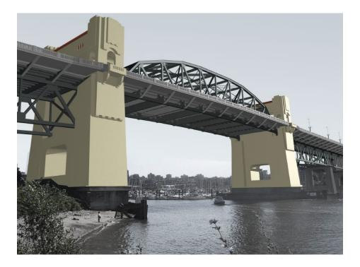
The second treatment must leave the main towers unchanged and will therefore require that the sidewalks narrow at these locations to create a "pinch point" (see right and below). This narrowing of the sidewalks must be designed to minimize conflict between sidewalk users.
