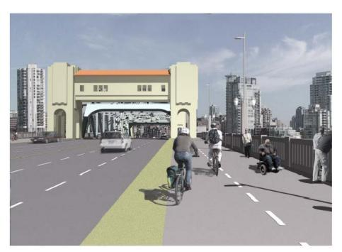
The 6.0m wide sidewalk treatment will apply for most of the length of the bridge. However, in at least six locations on each side (at the brazier towers at the north and south abutments and at Piers 1, 3, 4 and 6), the sidewalk must accommodate the existing structure in a different way.
