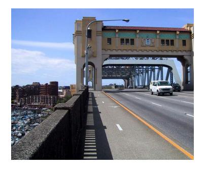
The proposed widened sidewalks will provide a minimum 6.0m usable width. The figure below shows a 1.0m clear zone adjacent to the curb, a 2.5m bicycle path and a 2.5m pedestrian path. The new sidewalk structure must be designed to accommodate other configurations (e.g. a curb-side railing, a 2.5m bicycle path and a 2.8m pedestrian path).
