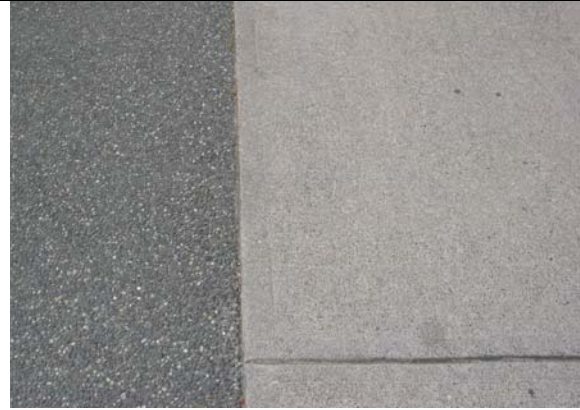
Figure 1a - Detail of Broom Finish Concrete with exposed aggregate concrete
