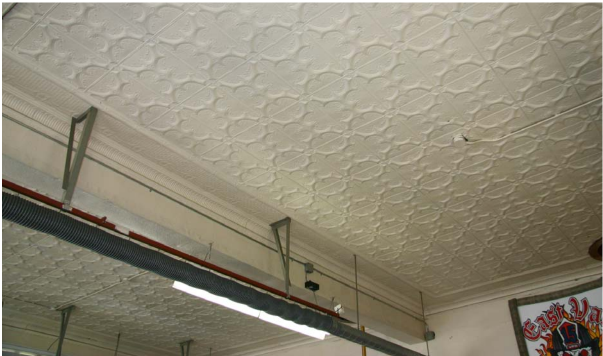
Truck bay ceiling
