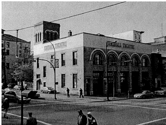
FireHall Theatre – listed as 'B(M)' on the heritage inventory is an example of adaptive reuse of a firehall building
