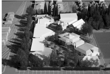
Model View Looking at Campus from the West - Full Development Envelope Shown
