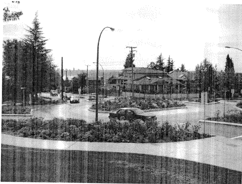
Figure 4 - Modern roundabout in North Vancouver
