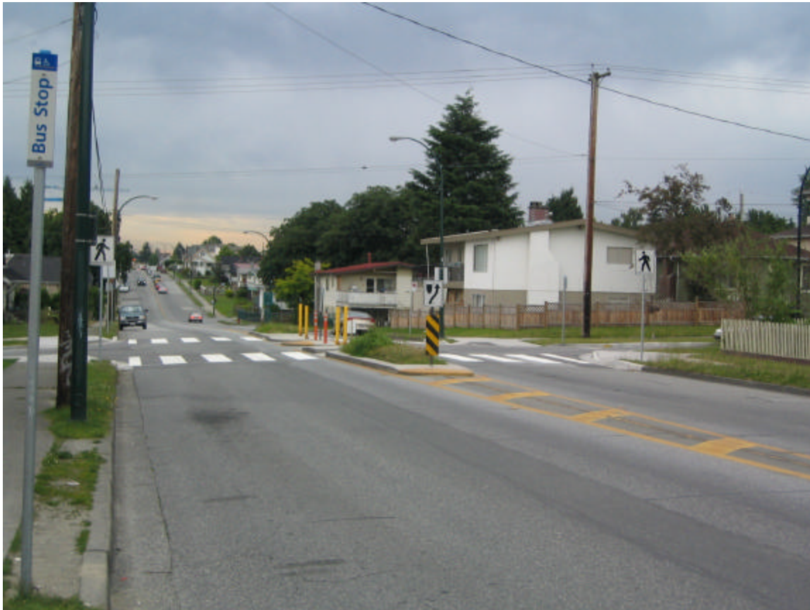
Figure 1. New crosswalks on 25 th Avenue at Windsor Street
