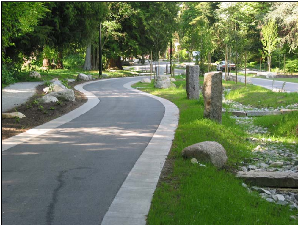
Figure 1. Crown Street Phase One, May 6 2005.
