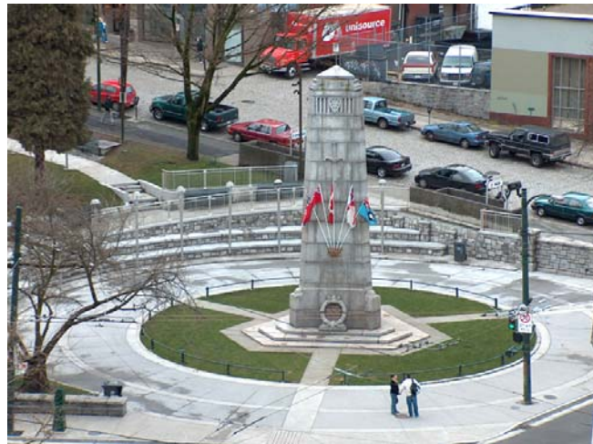
Figure 7: Victory Square Park Renovations
