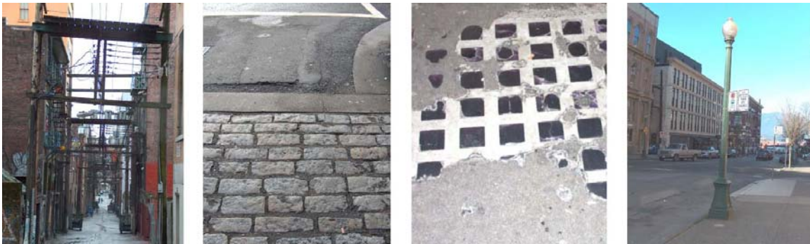
Figure 8-12: Alley H-Frames; Hamilton Street Paving; Areaways; Lamppost
