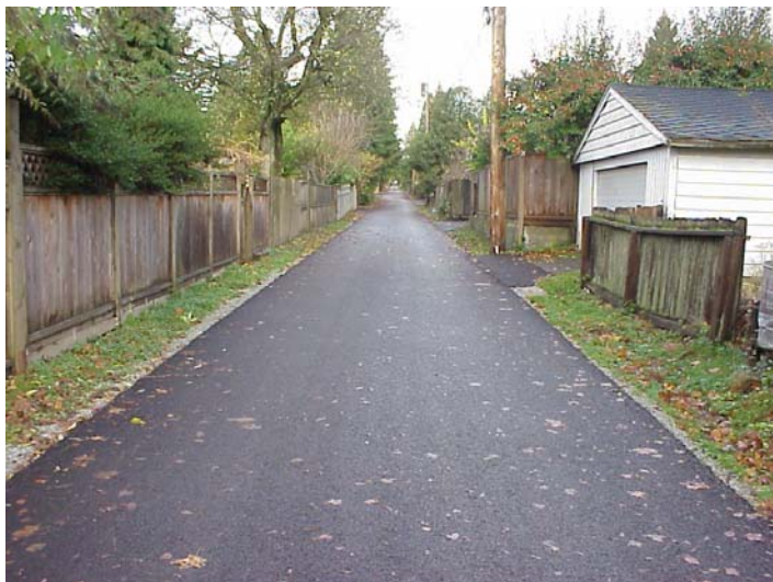
Photograph of One of Vancouver's Existing Center Strip Lane Paving Projects
