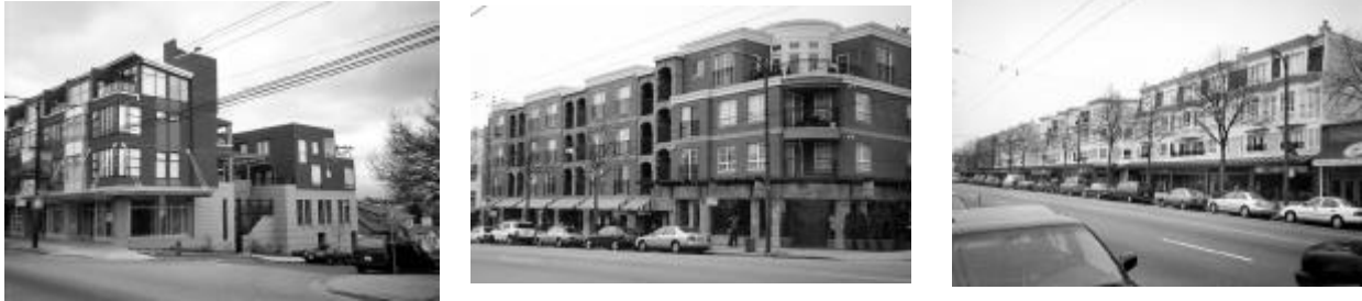
Figure 19. Examples of of stucco, brick, and vinyl siding used well
