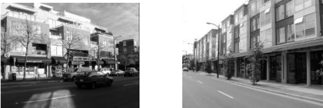
Figure 21. Examples of architecturally integrated, high quality awnings and canopies
