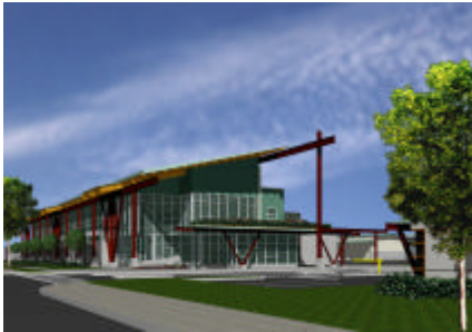
Figure: The City's new LEED Silver rated City Works Yard building
