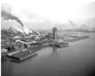
Figure: Older polluting industry around False Creek
