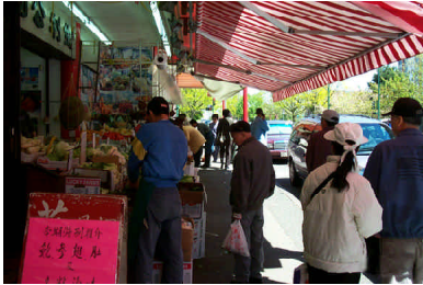
minimum pedestrian clearance compromised (previous)
