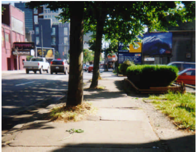
poor sidewalk conditions
