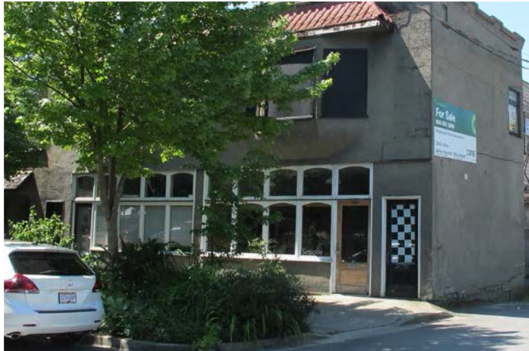
Photo 1: 2655 Maple Street Looking South-West From Maple Street (circa 2016)
