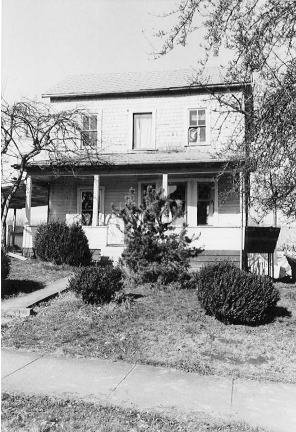
Photo 3: The Emily Durie House (looking north), 1970s or 1980s. At this time the house was still in nearly original condition. Note that the centre upper floor window had been removed.
