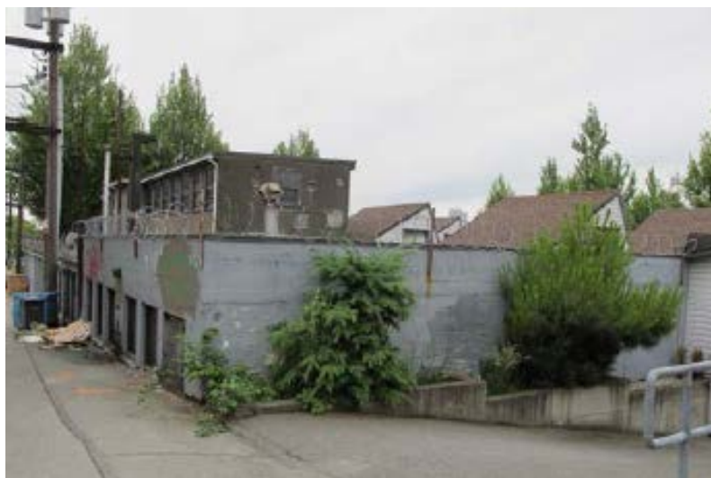
Photos 8 and 9: West Side (top) and East Side (bottom)
