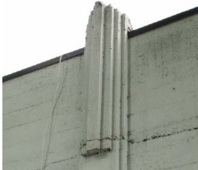
Photo Collage 1: Concrete Details
