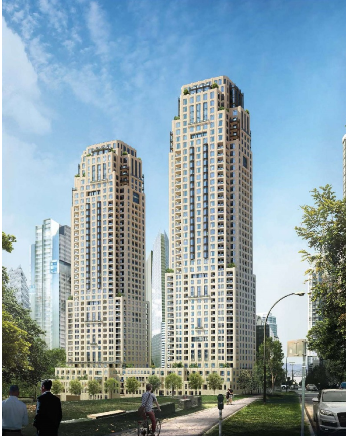
Figure 1: View from Robson Street
