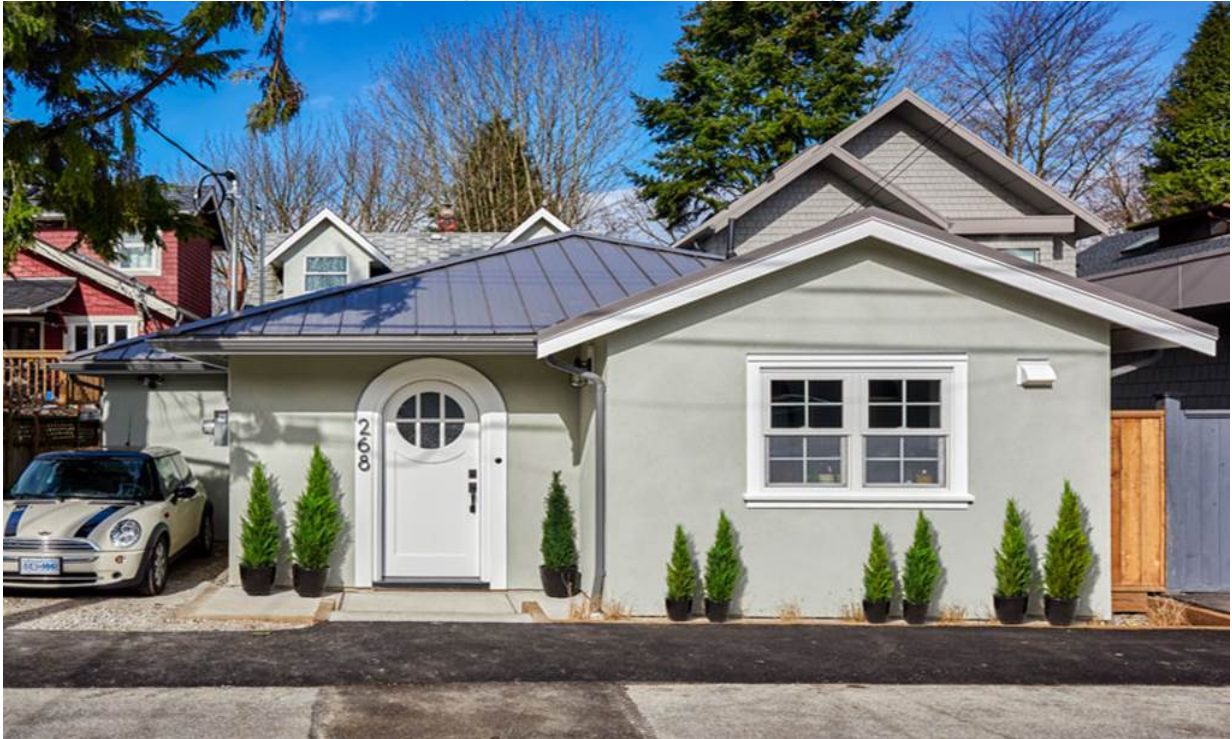
Figure 7: Example of a one-storey laneway house 5
