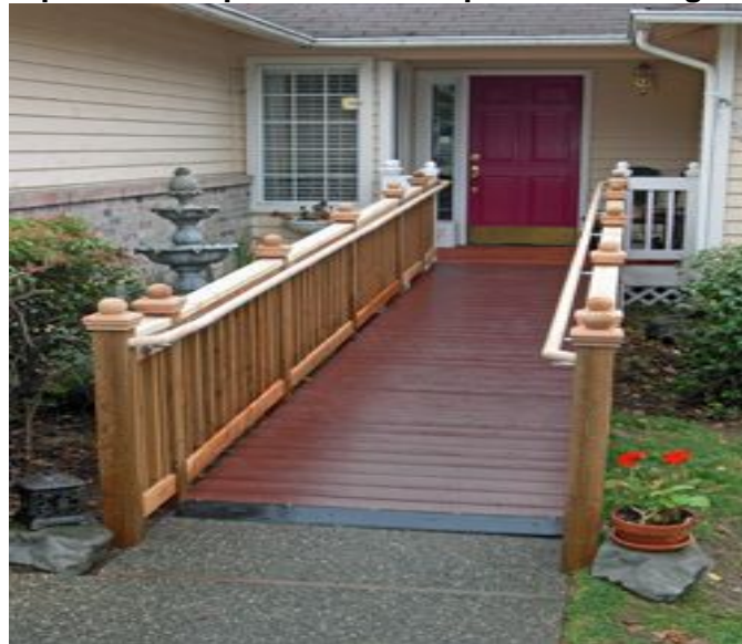
Figure 6: Example of a ramped accessible path into a single-family house 4
