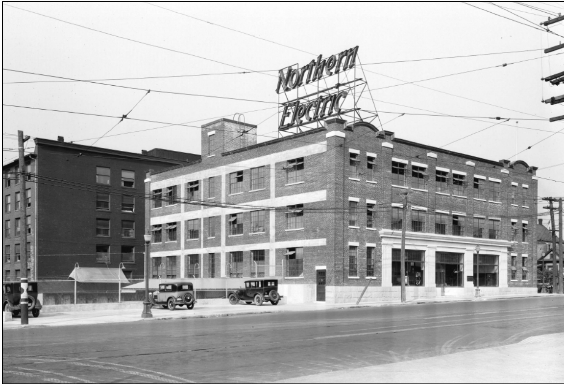
Figure 6: Historic Photo of the Northern Electric Company Building showing the 1928 phase
