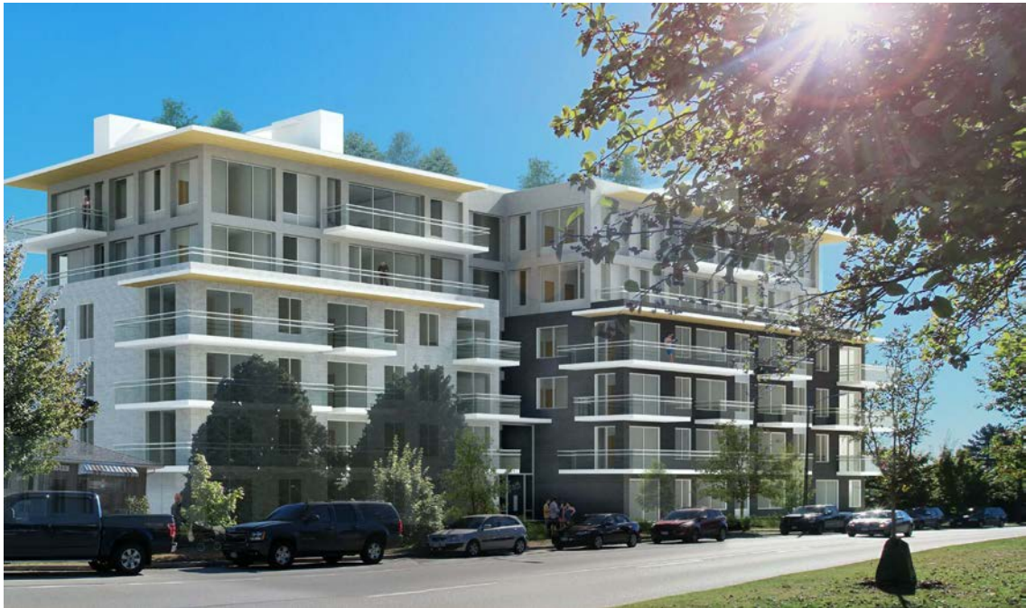
Perspective on Cambie Street (looking southwest)
