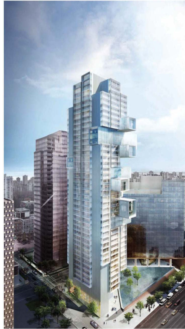
Aerial View from East
