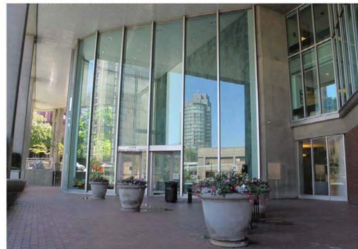
Exterior View of Lobby
