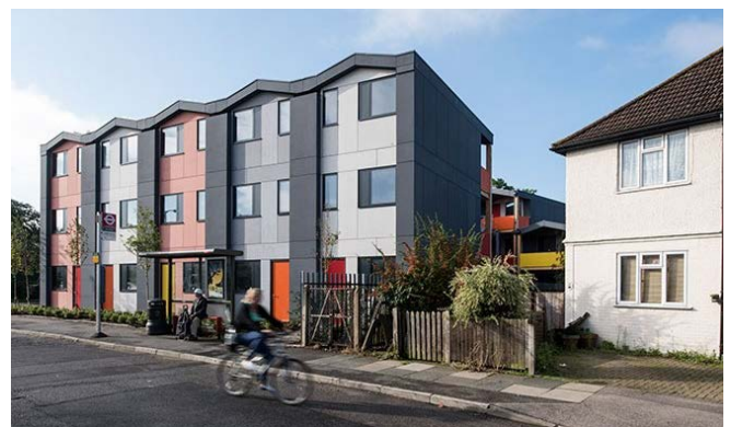
TMH development should respect predominant street patterns (Y-Cube Temporary Housing, UK) Photo: TBD
