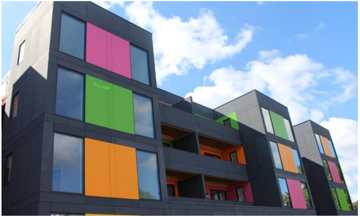
Bold colours, window detail and balconies animate façade (Lewisham Family Housing, London) Photo:TBD
