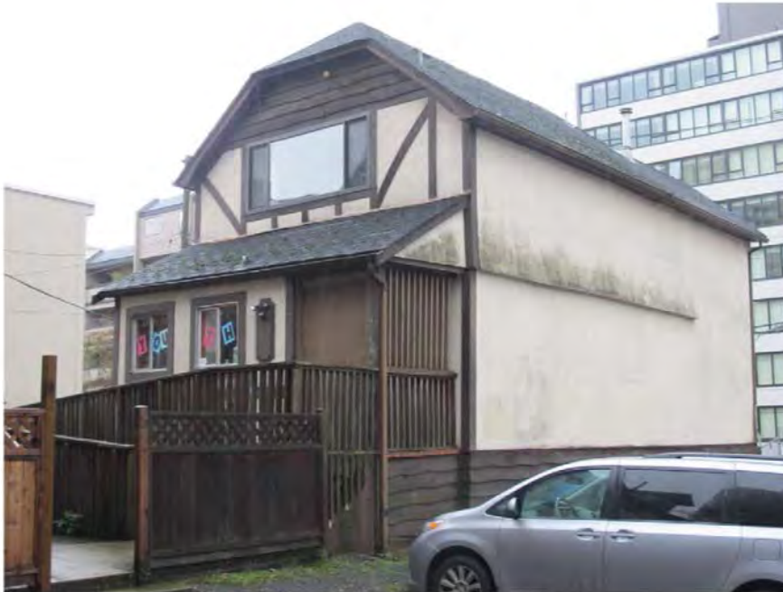
1023 Nelson Street front façade (facing south)
