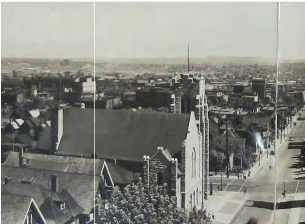
First Baptist Church, view from Nelson Street, 1936 [City of Vancouver Archives 371-3177]
