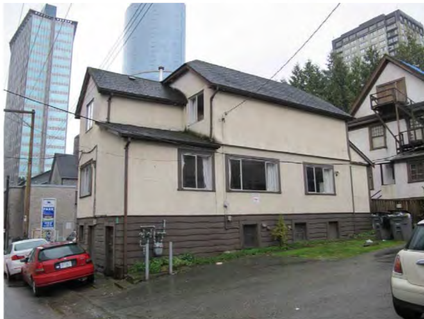
1023 Nelson Street west elevation
