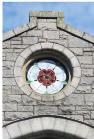
Pinder Hall east elevation
