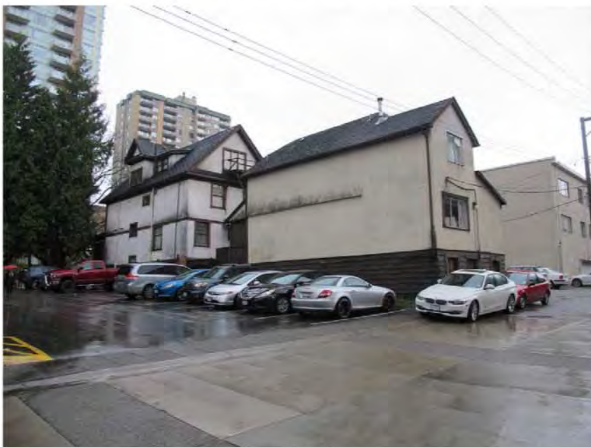
1021 and 1023 Nelson east elevations
