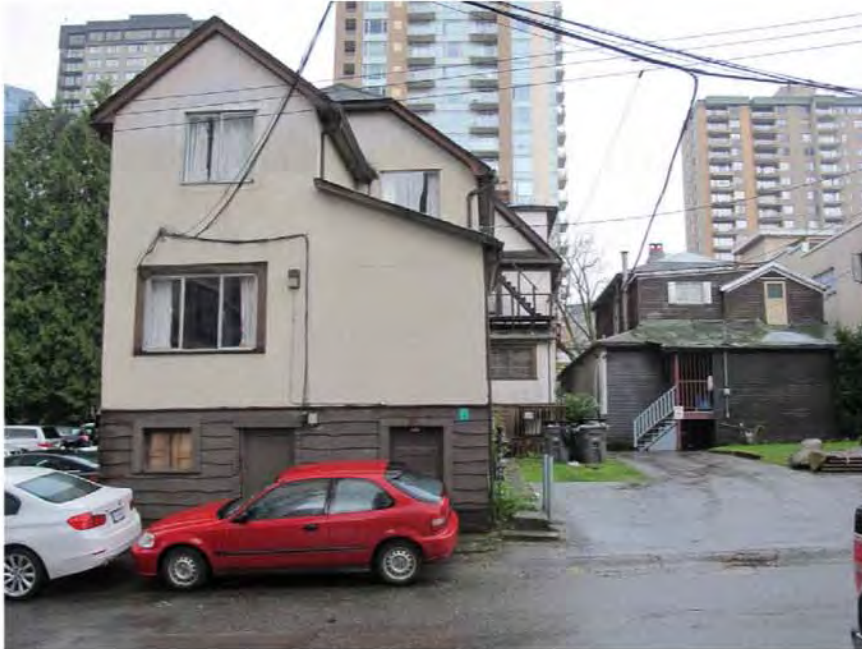
1023 Nelson Street rear elevation
