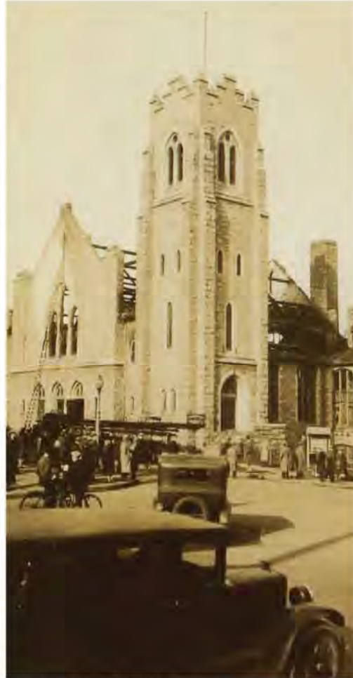
The aftermath of the First Baptist Church fire at Burrard and Nelson in downtown Vancouver [Bentall, The Charles Bentall Story , page 112]
