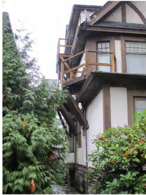
1021 Nelson Street west elevation
