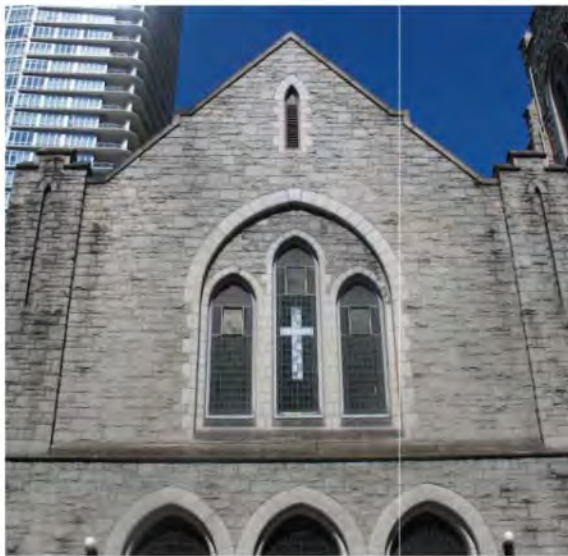
Sanctuary south elevation
