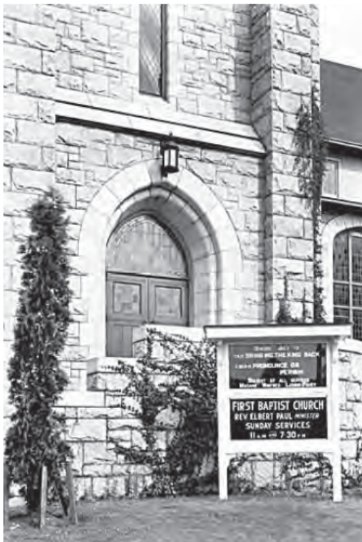
First Baptist Church Doorway and Sign, 1936 [Vancouver Public Library 8106]
