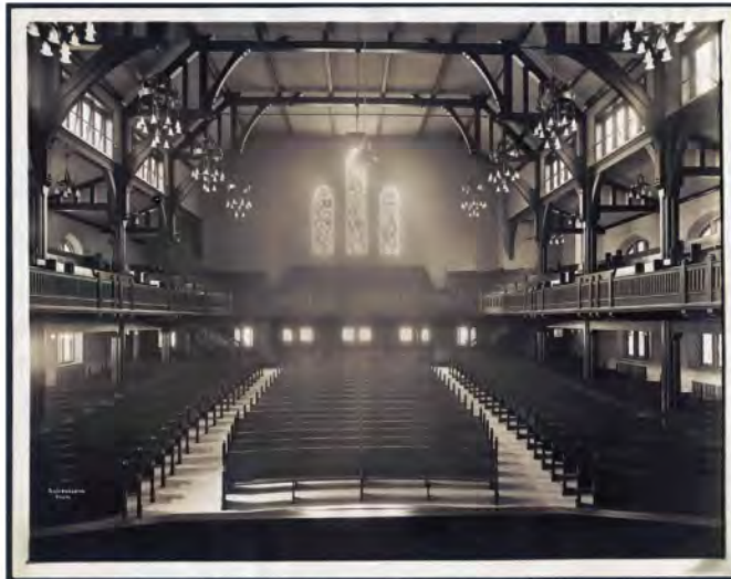
First Baptist Church sanctuary [Horwood Collection, Archives of Ontario]
