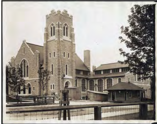
First Baptist Church, construction nearly complete [Horwood Collection, Archives of Ontario]
