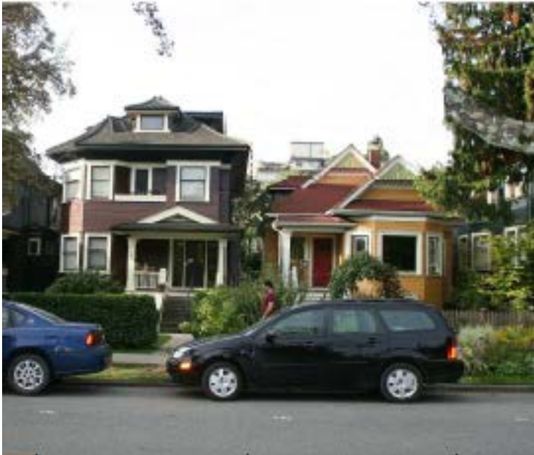
Existing Front of 1150 Comox Street
