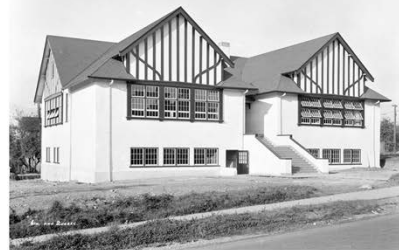
Simon Fraser Annex, 1930
