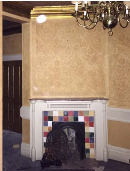
Main floor fireplace and crown moulding
