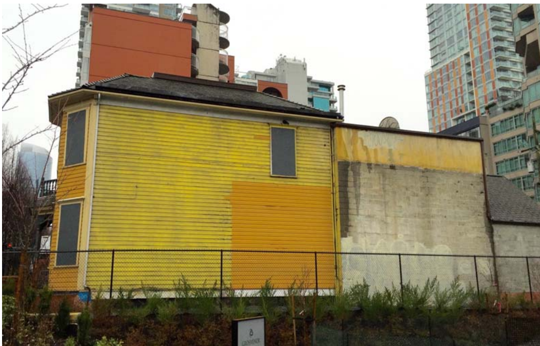
South elevation, 2015; original channel siding is shown on historic part of Leslie House, plus recent repair to entry to former Il Giardino restaurant. Concrete additions replace the original single story wing
