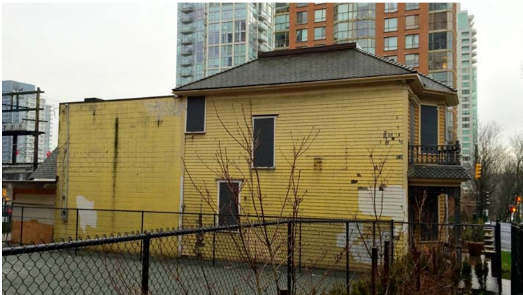
North Elevation, 2016; wooden shingles cover the original channel siding; coloured glass window can be seen in this view.
