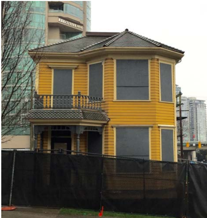
January 2016; note windows have been boarded for security
