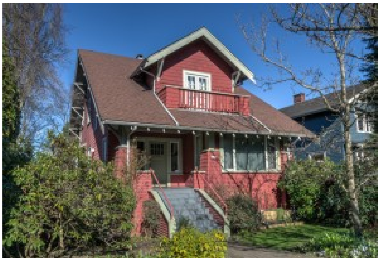
Photo 1. 4255 West 12 th Avenue - front elevation
