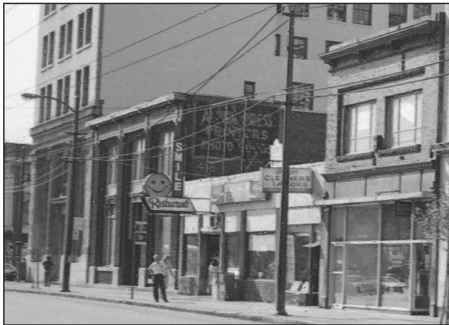
Partial view of a 1981 photograph of the 400 block of W Pender. By the 1970s the cornice had been lost. The Smile Restaurant's sign no longer survives. Vancouver Achives CVA 779-E10.22
