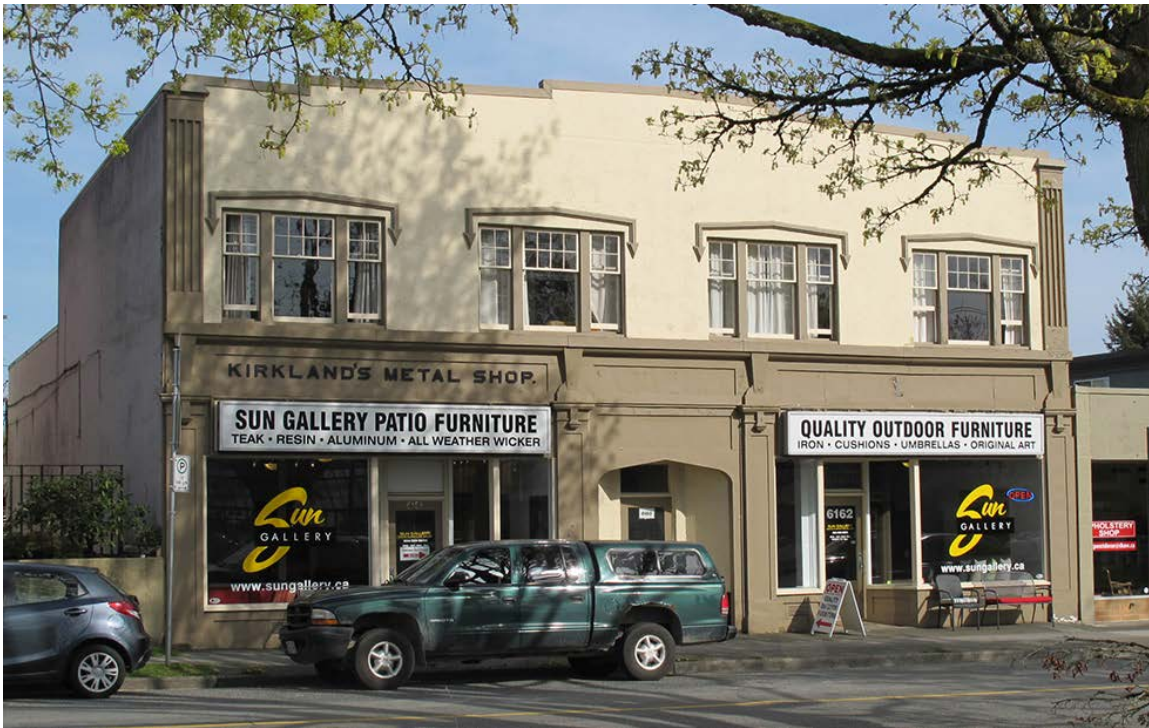
Photo 1 : West Façade of Kirkland's Metal Shop
