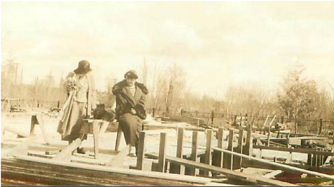
Photo 8: The Wilmar Residence under Construction (circa 1925)
