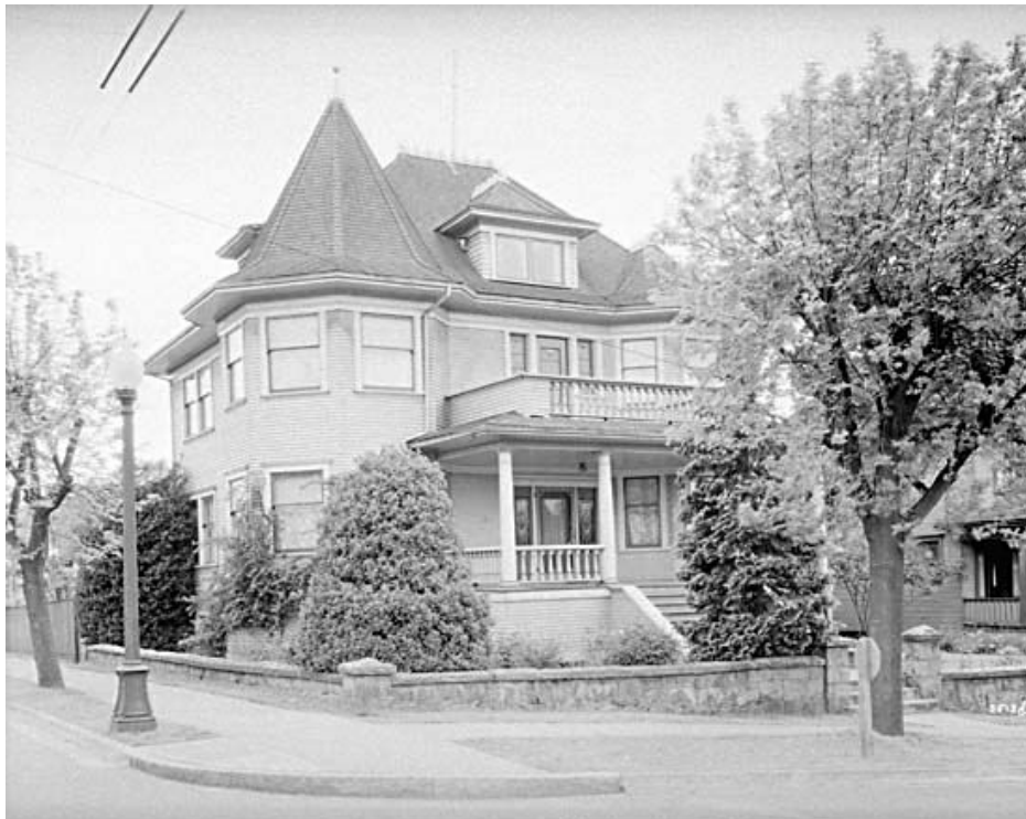
Figure 2: The Brookhouse Residence (circa 1932) looking southwest from Parker Street and Victoria Drive
