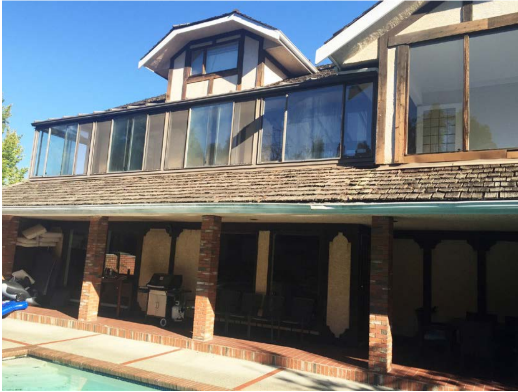
Photo 3. Partial South Elevation
