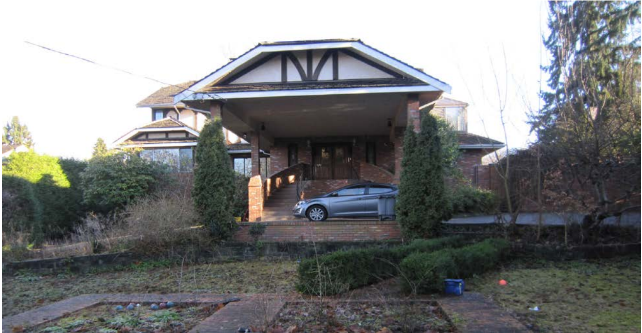
Photo 1. Front Elevation (facing West)
