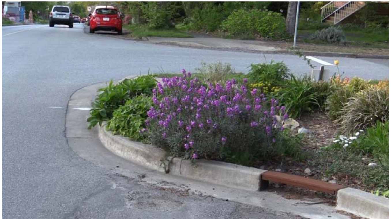
Existing Infiltration Bulge in Vancouver
