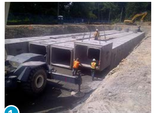
UBC Detention Tank Installation
