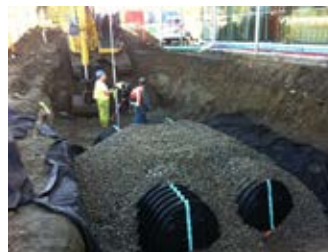
Infiltration Chamber Installation, MEC North Vancouver
