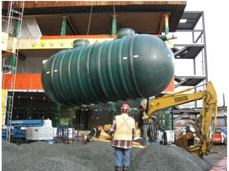
Detention Tank Installation, MEC Head Office
