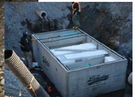
Copper Valley Oil Interceptor installation (Photo Credit: Langley Concrete)
