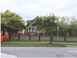
Existing Residence on Lakewood St.
