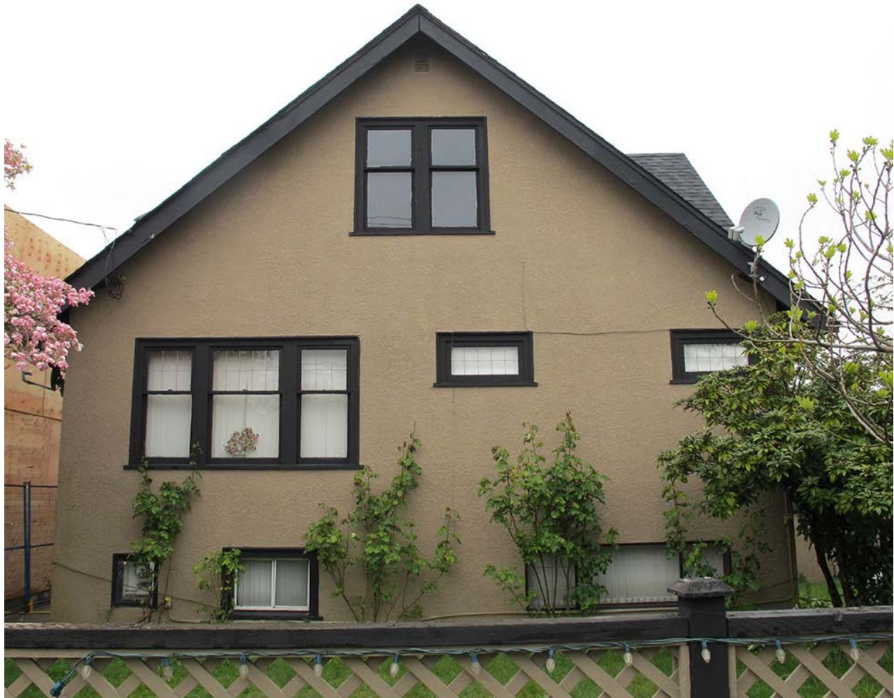
Photo 2: East Elevation of 2088 Charles Street
