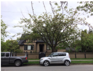
Existing Residence on Charles St.
