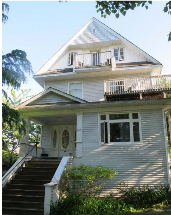
Photo 1: 1106 West 15 th Avenue - Front - Looking South (2015)
