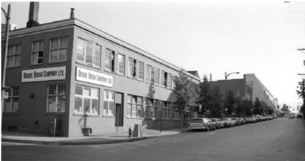
The Brodie Brush Co. Building photographed in 1981, the last year of the company's operation at this location. Since the previous photo from 1941, the building has been painted in a darker colour; expanded (back in 1942); and the windows on the upper floor, as well as a few on the ground floor on the Cambie Street elevation have been replaced. An additional street level entry has been opened on the Cambie elevation. credit: City of Vancouver Archives 799-E15.04
