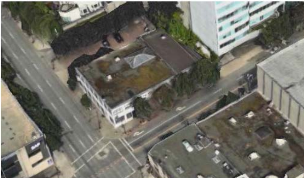
The 1942 extension is still visible in a current satellite view of the building's roof. credit: google crome
