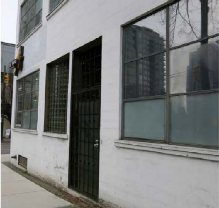
current view of reinforced concrete structure and concrete window sills
