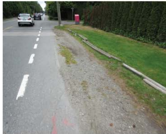
■ Poor pavement treatment
